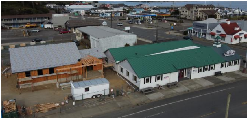
Drone view photo of construction by museum volunteer Pat Honstain.
