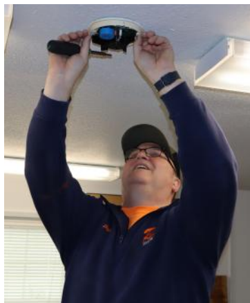
A technician from Reese Electric installs a new smoke detector. A grant from The Braemar Charitable Trust paid for security system upgrades.
